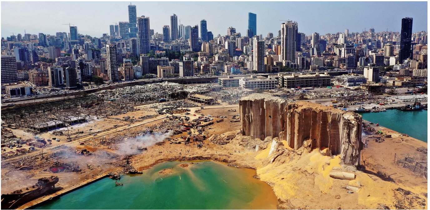
Beirut Port after the explosion caused by ammonium nitrate (4/8/2020).
