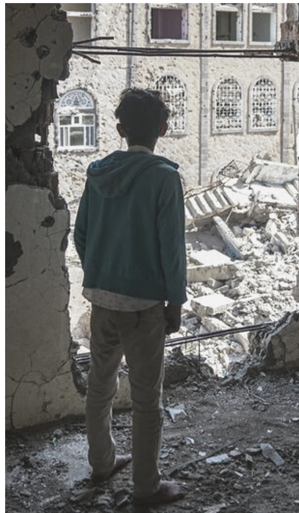
UNOCHA-Giles Clarke_A boy stands in the damaged interior of a building in Yemen.
